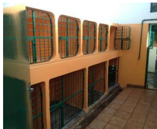
Kennels after refurbishment in Mozambique
